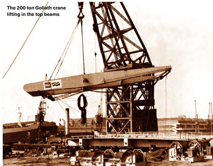
The deck being swung into position
