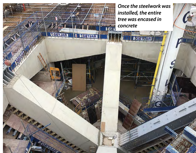
Tree two has a steel ring beam in order to create a void in the level four slab
