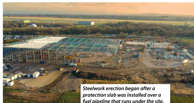
The crane's jib heights were restricted due to the proximity of the airport's runway.
