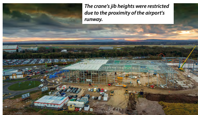
Steelwork erection began after a protection slab was installed over a fuel pipeline that runs under the site.
