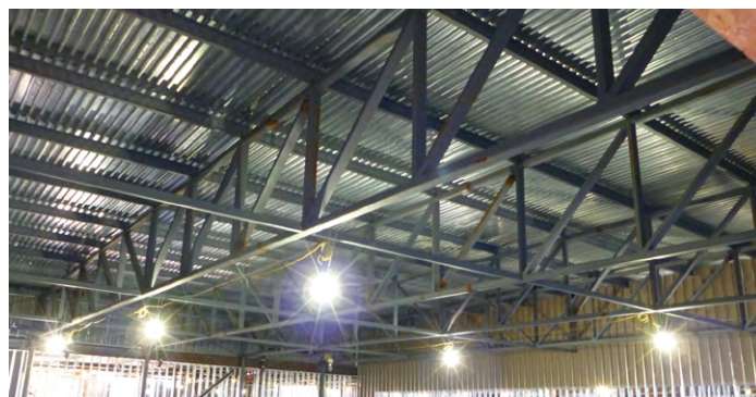
Figure 5.1: Top and bottom boom restraints
