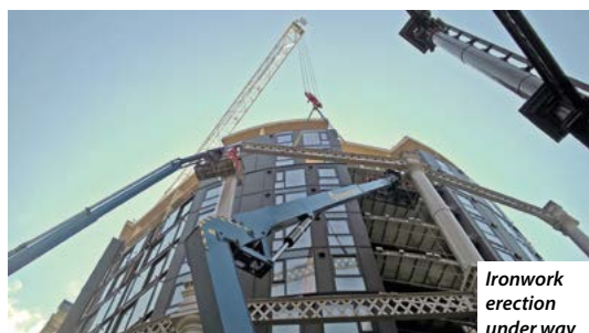
A 'rocket launcher' prepares to lift and position a column
