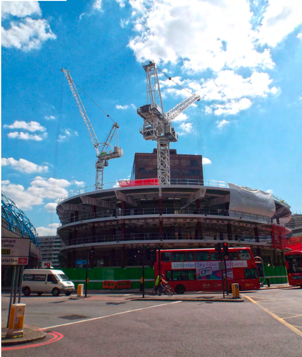
Deep trusses on the third floor support the residential tower
