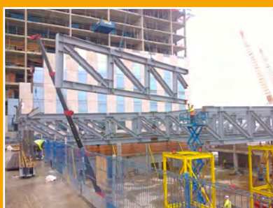
Temporary supports were set up to allow the trusses to be installed in three sections
