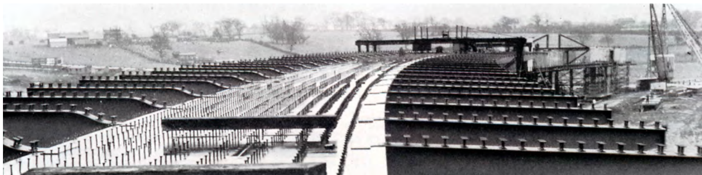
This illustration shows the top surface of the three-cell box girder or spine beam and the cantilevers forming the structural deck.
