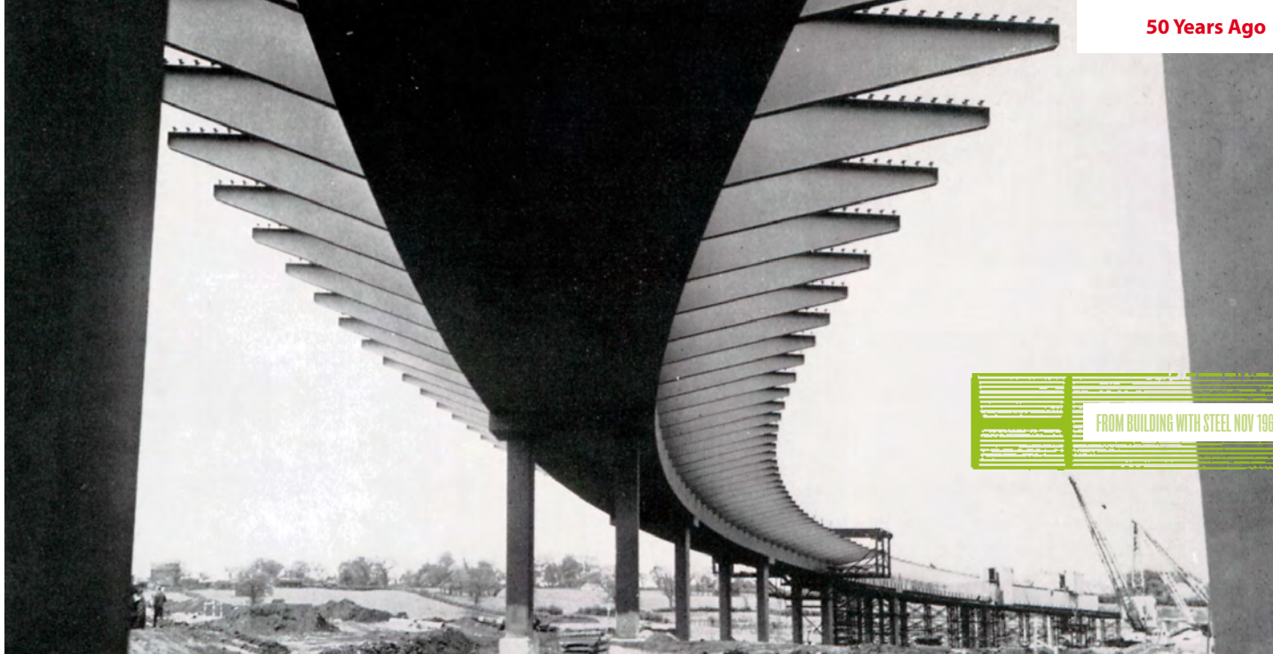
The underside of the viaduct, showing how the twin-tapered hollow box column piers support the spine beam and cantilevers.
