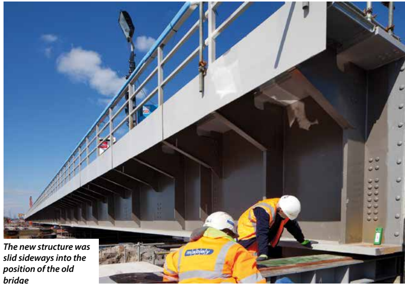
The bridge was launched in four individual sections
