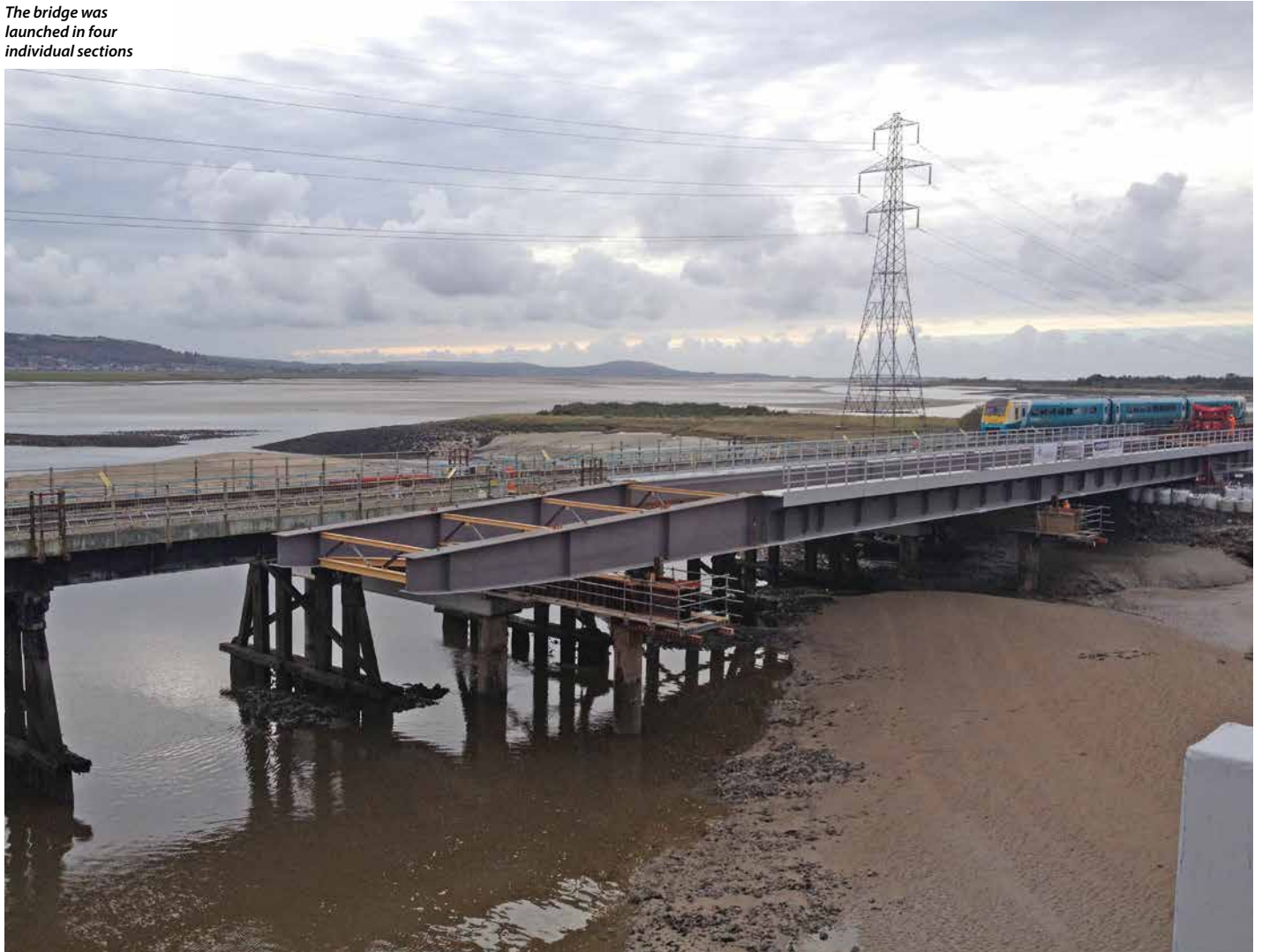
The new structure was slid sideways into the position of the old bridge
