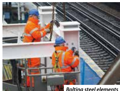
Bolting steel elements
