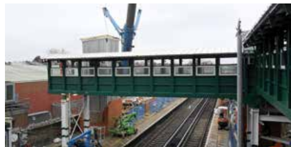
Above: A large bridge section is lifted into place
