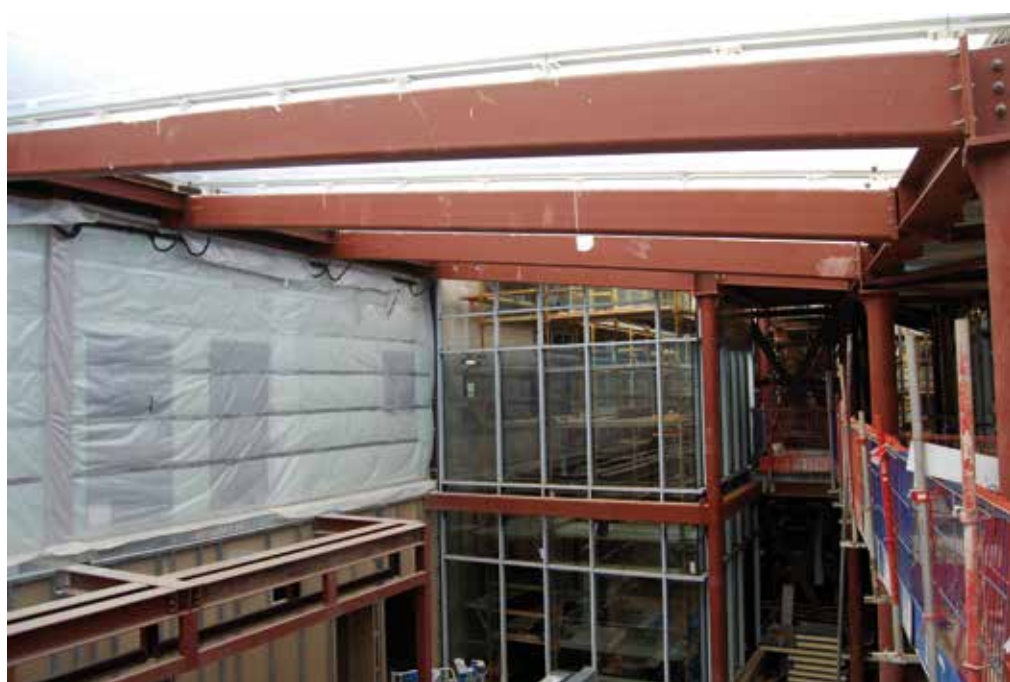
The steel structure wraps around a retained building once used as a granary
