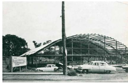
Above: Seen on the course of construction in the City of Dartmouth, Nova Scotia, is a bowling centre of structural steelwork exported from Britain. The building is 114 ft. in span by 11 ft. high to eaves and 117 ft. long.
