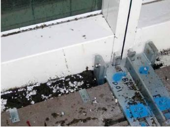
Figure 1 Bracket with serrated washers and T-bars in slots ©Yuanda Europe
