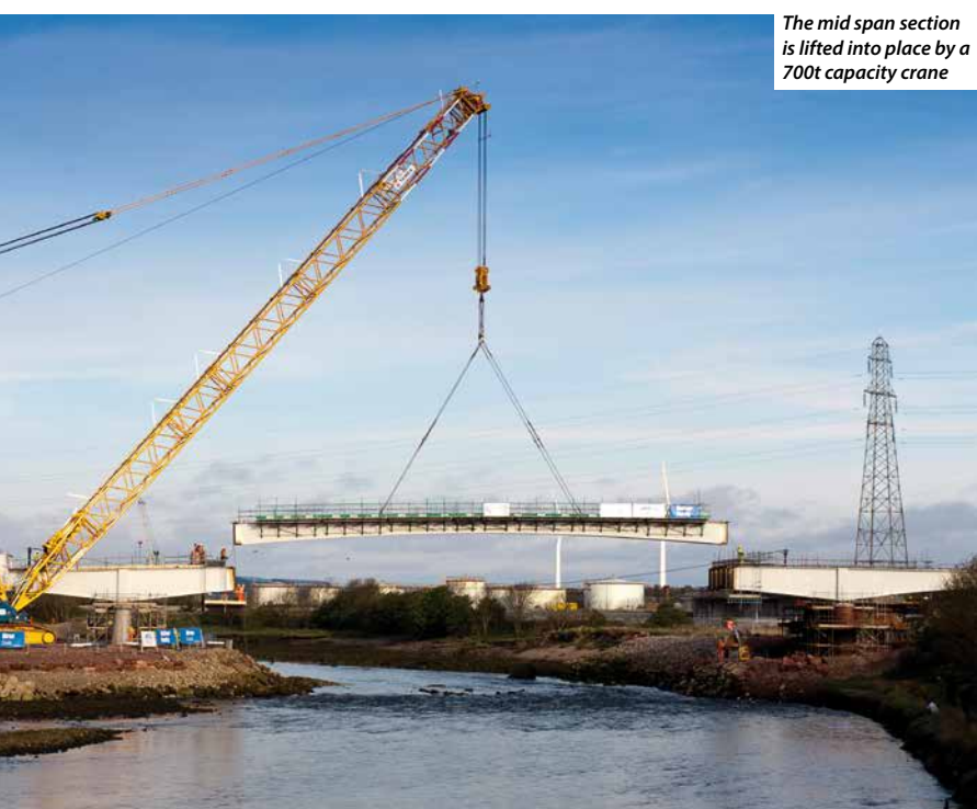
Steel was erected by cranes positioned on the river banks to avoid any work in or over the river
