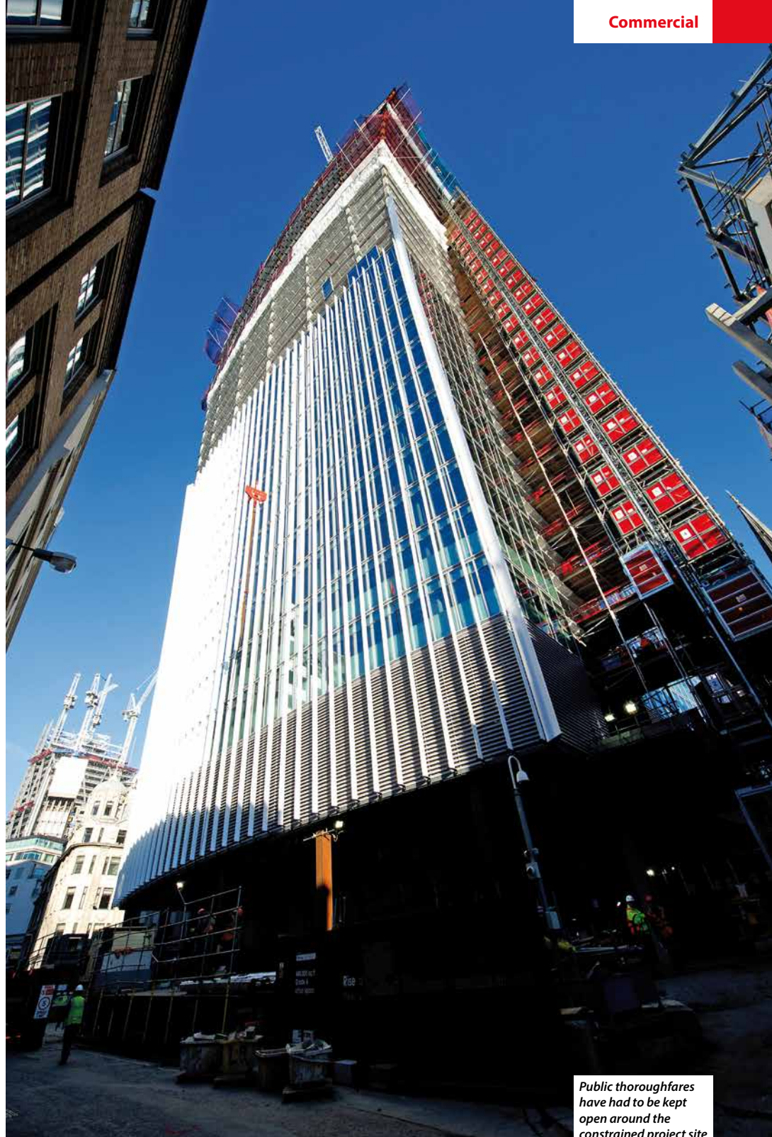
Many of the columns are faceted every two floors to create the building's shape
