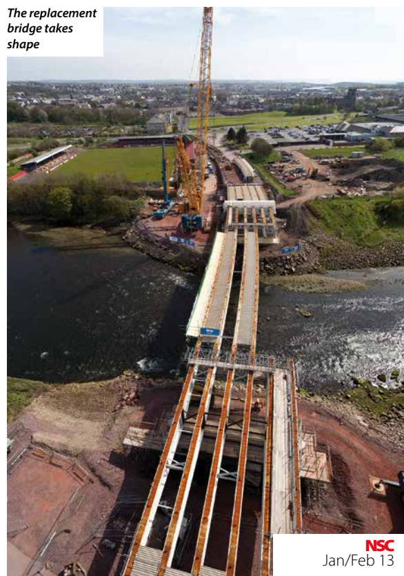
The mid span section is lifted into place by a 700t capacity crane
