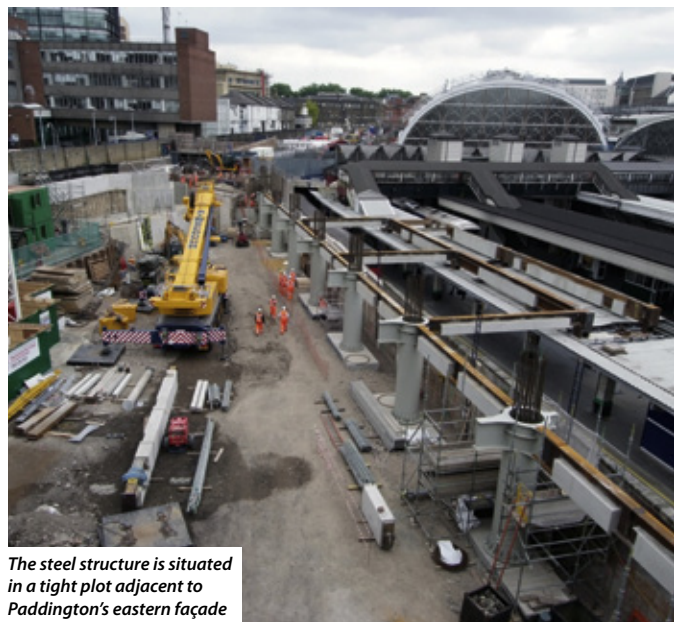
Tree columns will support the roof over the new taxi pick-up area
