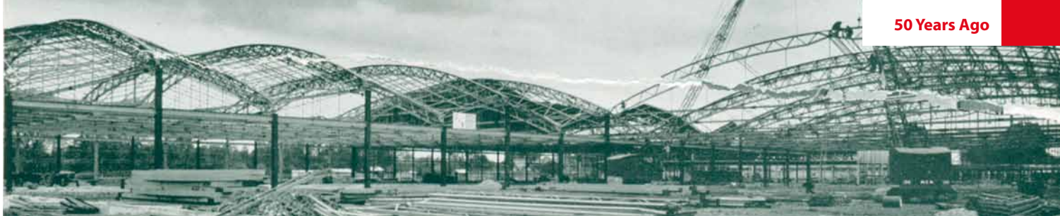
Structural steelwork for the machine and warehouse area
