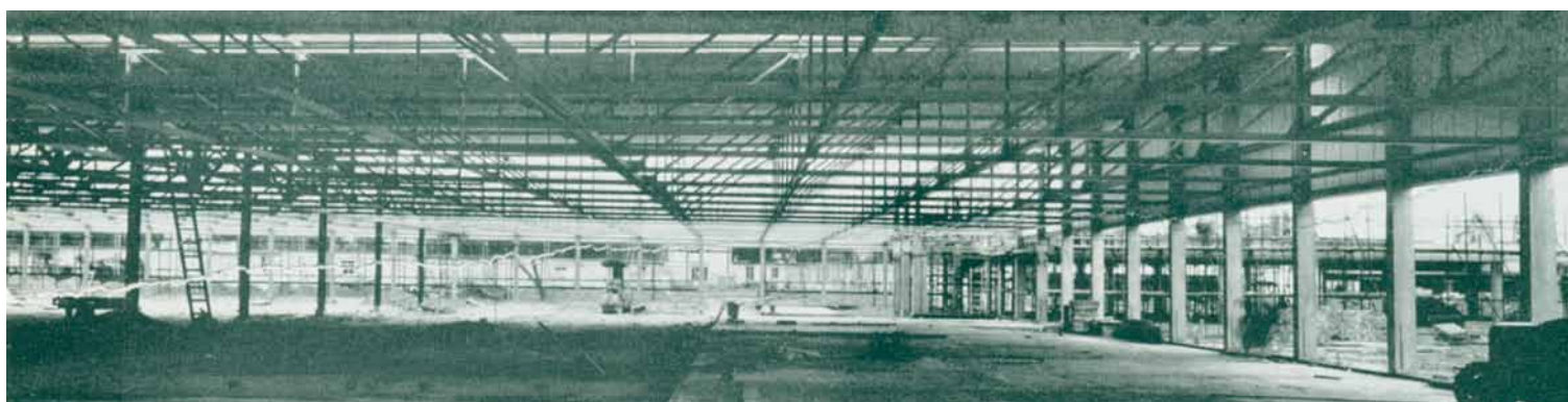
Interior of composition block, showing standard end trusses
