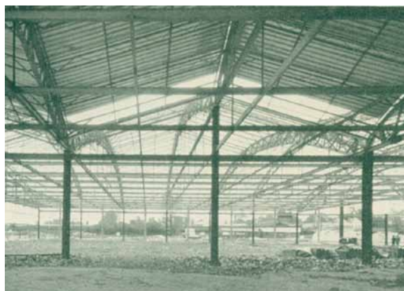
Interior of warehouse and machine block. Note the steelwork for the curved roof
