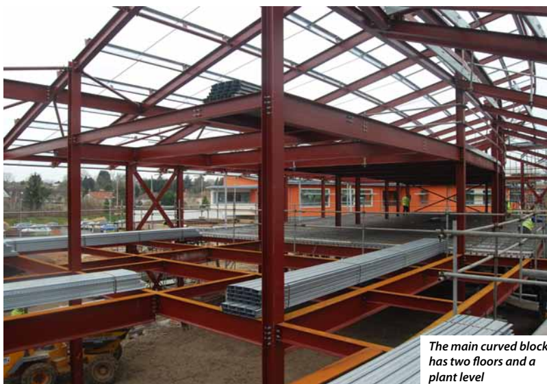
Curved members adorn the rear of each finger block
