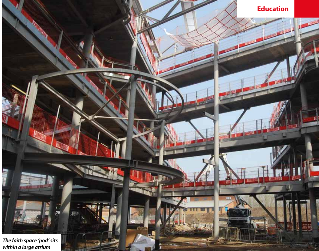
The structure's grid alters to accommodate a ground floor drama space
