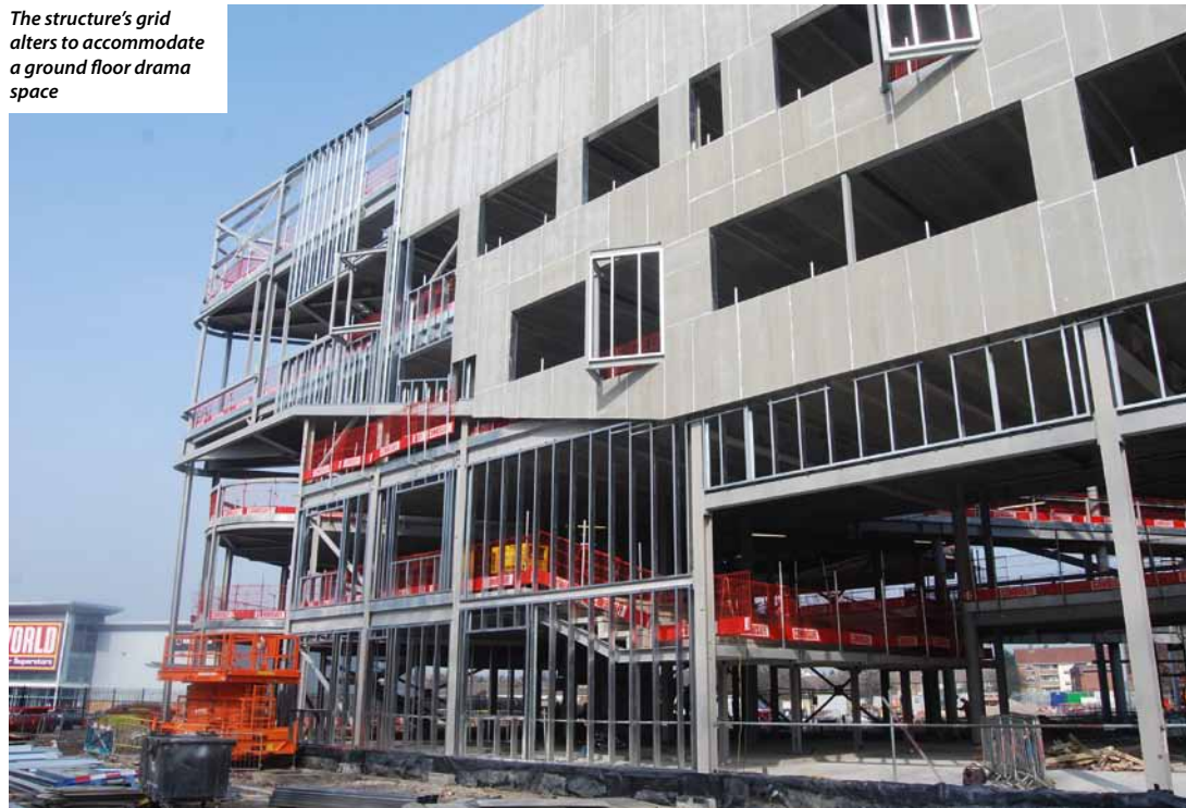
Warren trusses support the atrium's glazing
