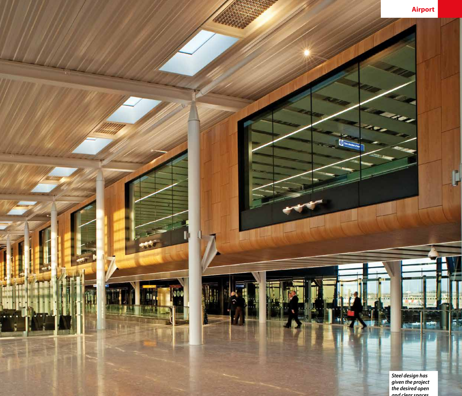
The seven passenger pods are braced and give the steel structure stability
