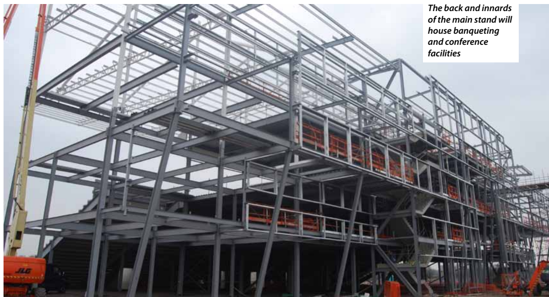
The main stand features a 39m deep cantilevering roof
