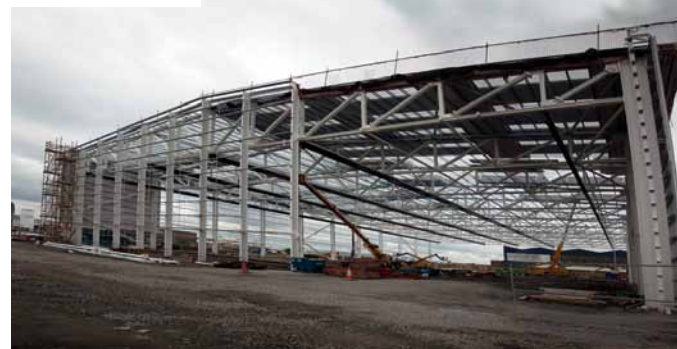
Roof trusses were brought to site in three separate segments
