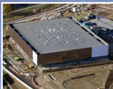
Steel's inherent sustainability and flexibility has come to the fore on the Olympic Park's Handball Arena. Already completed, the venue - which contains 1,000t of structural steelwork erected by Watson Steel Structures - will seat up to 7,000 spectators and host qualifying games for the handball competition as well as modern pentathlon fencing and goalball during the Paralympic Games. After the Olympics, the sustainable arena will become a multi-sports venue with retractable seating for around 6,000 spectators and flexible facilities catering for training and competition for all levels of indoor sport.
