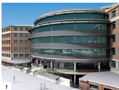
The completed rotunda (1) will house a new entrance hall (2) and the structure features CHS columns (3) which will remain exposed
