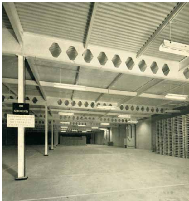
Right: Raw materials store. Note the extensive use of castellated beams.
