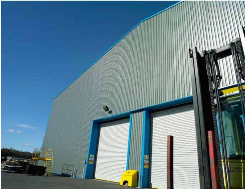
Figure 2: SolarWall® on the southern elevation of CA Groups own Profiling Mill in County Durham
