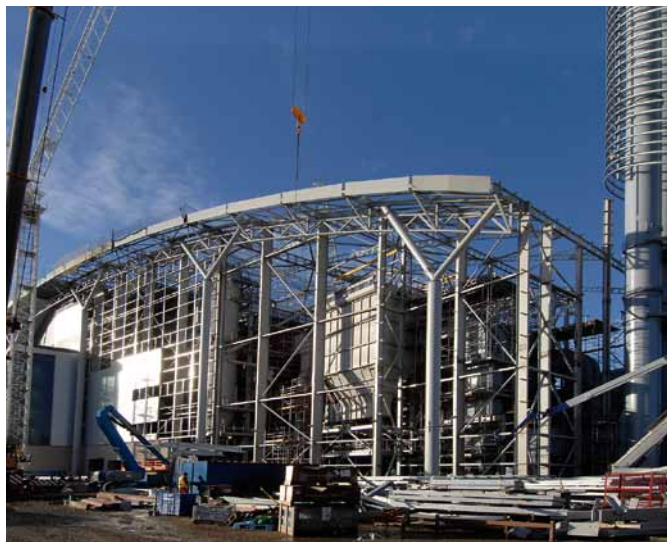
Energy from waste facilities require steel frames for the majority of their buildings
