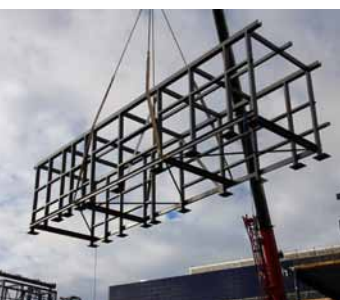
Below: Fully assembled modules were brought to site for the train enclosures
