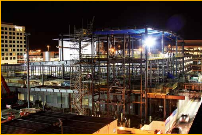
Above: The main structure is a portal frame design with three main spans of 20m
