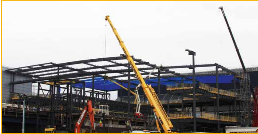
Above: The main structure is a portal frame design with three main spans of 20m
