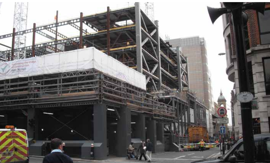
Top: Impression of completed structure showing an X-frame positioned on the cantilever Above: Minimal temporary works are in place at the station entrance Below: An hourglass structure is positioned inside each core to help stabilise the new building
