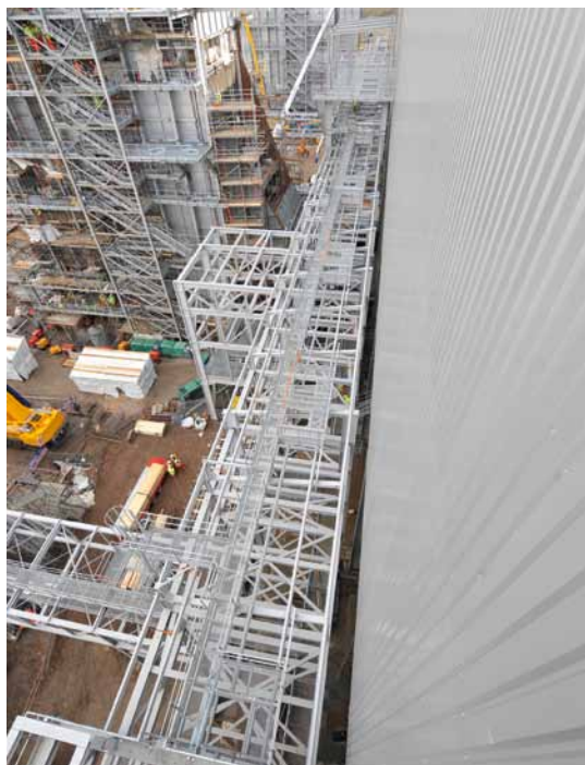
Above: A pipe rack connects each turbine hall to a substation
