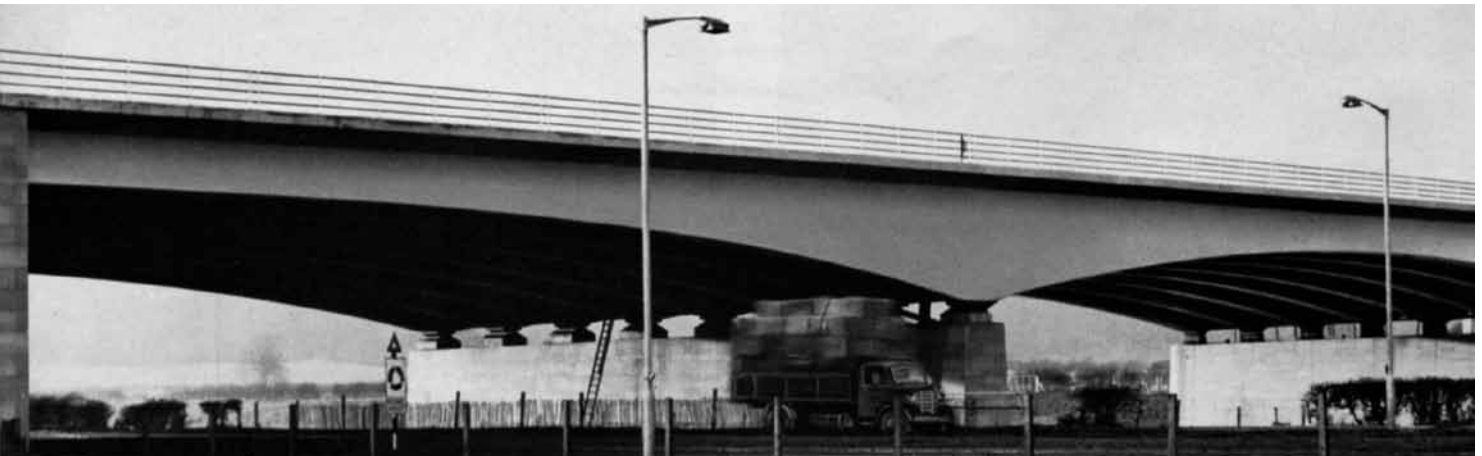
Above: Samlesbury Bridge spans the River Ribble on the Preston By-Pass. It is an all welded structure with two 120 ft side spans and a 180 ft centre span.
