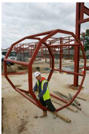
Below: One of the project's three roof lanterns is assembled
