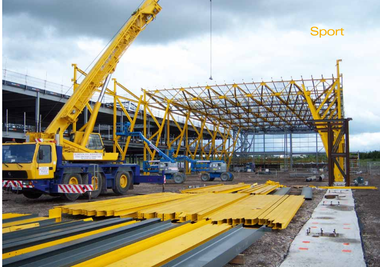
Above: Using the spine building for temporary stability, trusses are erected to form the athletics hall
