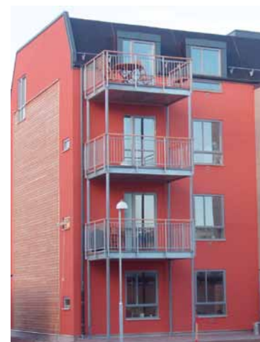
Figure 2: Independently supported balconies to minimise thermal bridging
