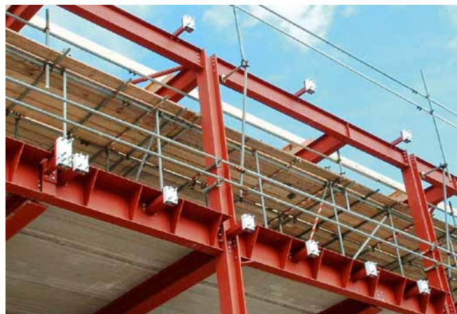
Figure 3: Isokorb thermal break units attached to steel frame
