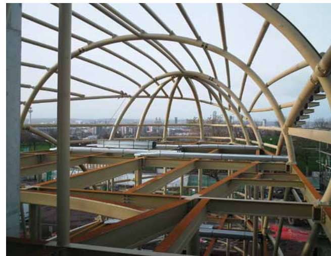
Above: Steel ribs form the arc of the handle's shape.
