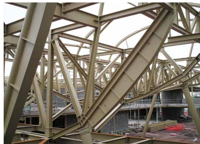
Below: A series of bowstring trusses support the handle.
