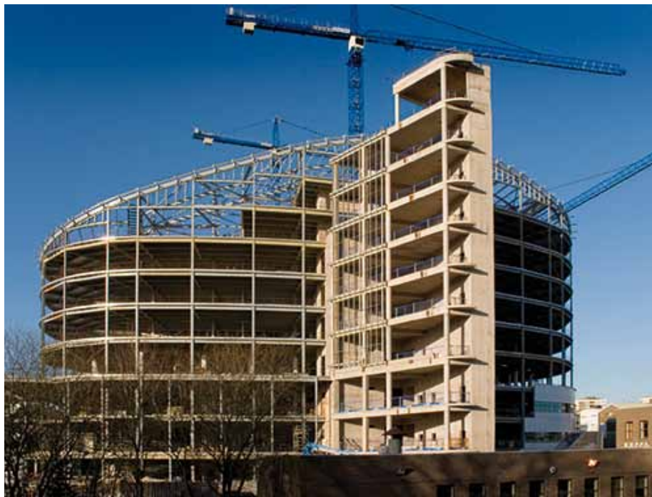
Right: The three pods are linked by slipformed concrete cores.
