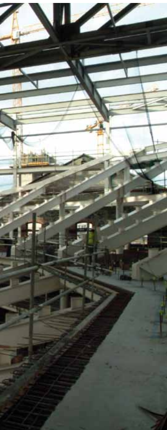
Below: The Dublin O 2 project extensively used offsite application of intumescent coating.
