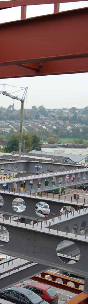
Above: Braced cores provide the stability for the extension.
