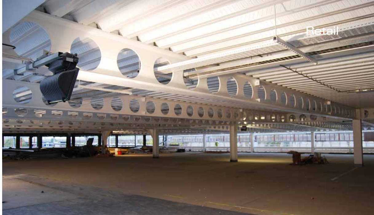
Above: Cellular beams will allow more light into the large car park, especially at night.
