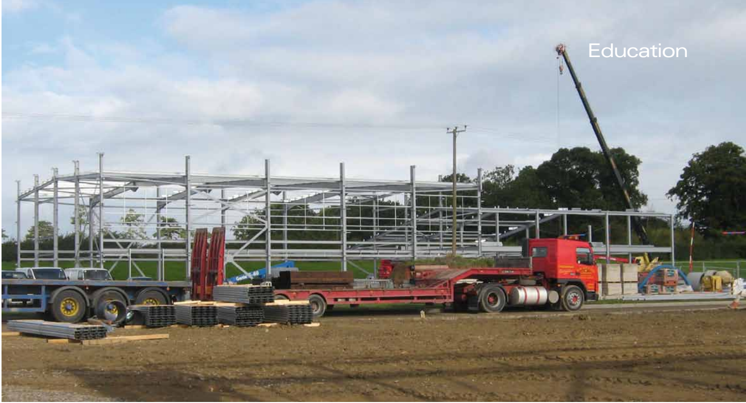
Above: Cauntun erected 800t of structural steel during a three month programme.
