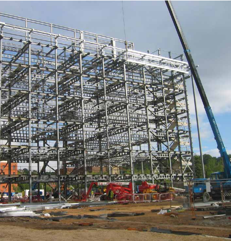
Above: A steel frame was chosen for its speed of construction. Right: Feature architectural elements adorn most facades. Below: One elevation has a large weathering steel facade. Left: The building is cube-shaped as this offers the best way of regulating its internal climate.
