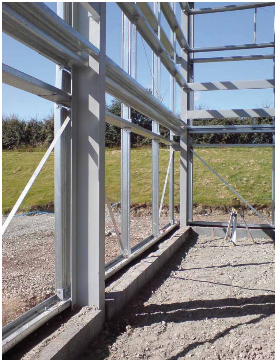
Below: A steel frame was chosen for its time and flexibility advantages.
