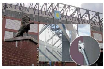
The new Aston Villa Football Club signage, atop the team's Trinity Road stand, was recently fixed into place using the Lindapter bolt-on CF high friction clamp. The system allowed the lettering - which is two metres high, 50m wide and mounted on to two channel sections - to be bolted onto the stadium's structural steelwork without any drilling or welding.
