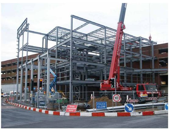
A shopping centre extension, spanning bus lanes and a main arterial road, has required a phased steel erection programme in order to keep the highway partially open to traffic throughout construction.
