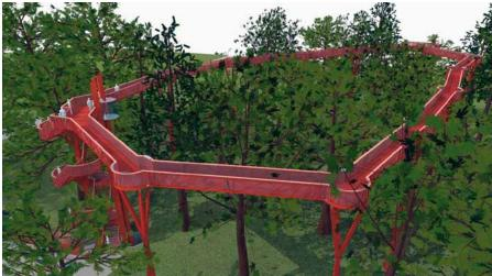
Britland started the erection process just before Christmas and expects to complete the job by early March. The process involves setting the pylons in place first - four supporting most of the node platforms and six for the larger classroom - and then lifting the walkway sections into place between the nodes.
