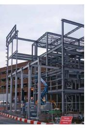
Above: Feature CHS columns will be filled with concrete for extra impact resistance.
