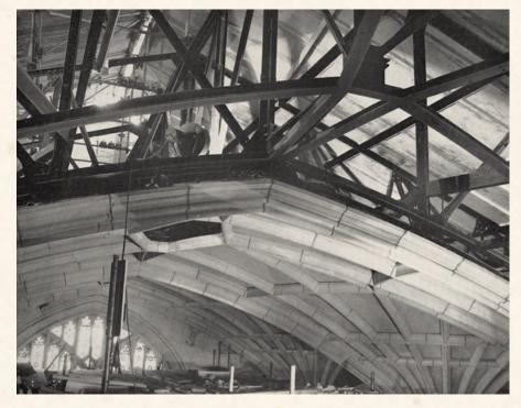
roof and a scheme for its repair or reconstruction in timber. This was done but subsequently rejected on the score of high cost and slowness of execution. There was also the difficulty of insuring against continued beetle infestation.
