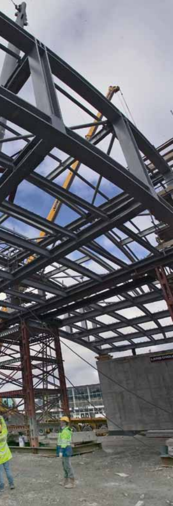
Above: The curved bridge was assembled in five sections.
