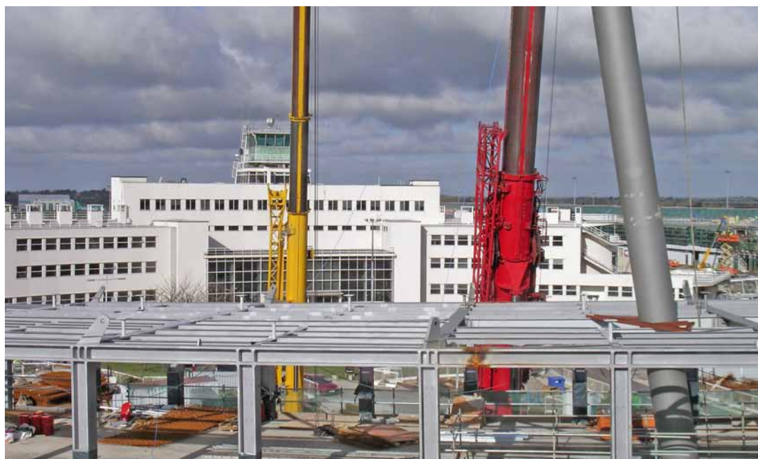
Above: The curved bridge was assembled in five sections.
