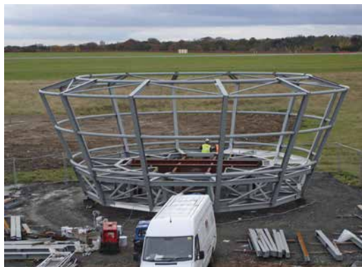
Above: A tubular CHS framework will form the curved profile of the tower.
