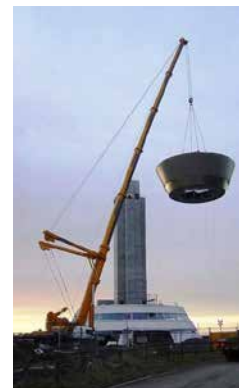
Above: A tubular CHS framework will form the curved profile of the tower.
