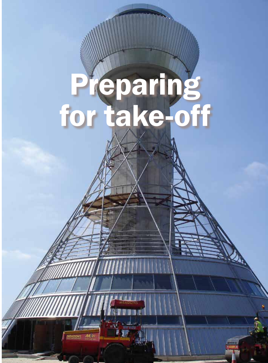
Above: A tubular CHS framework will form the curved profile of the tower.
