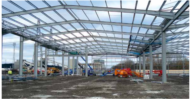
Above: Lafarge required long column free spans for its warehouse.
