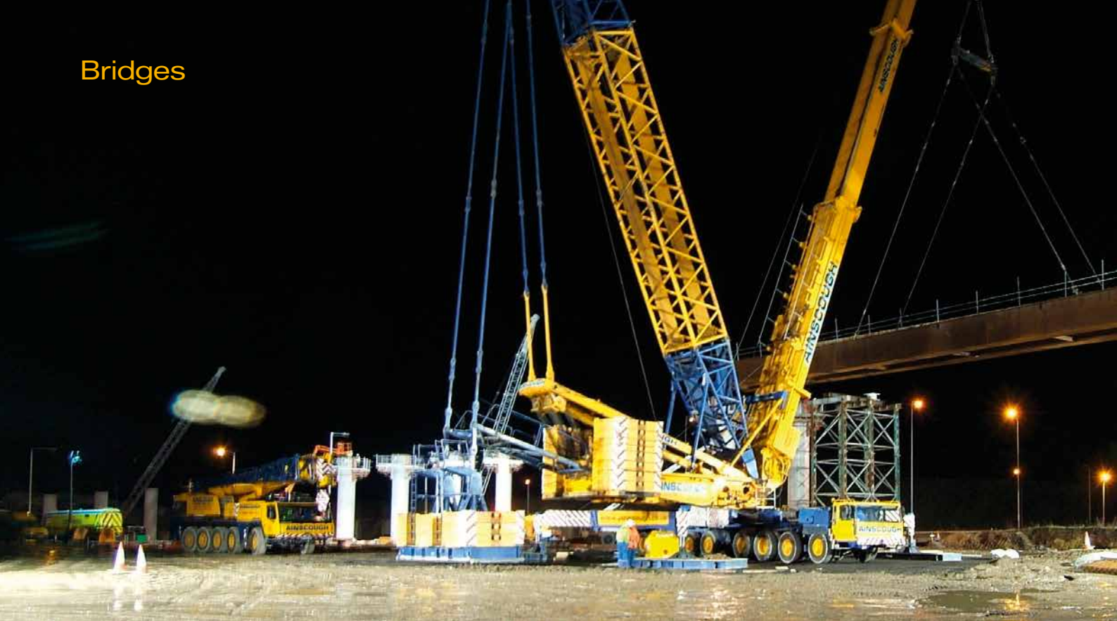
Above: the majority of steelwork is lifted by one 1,000t capacity crane.
