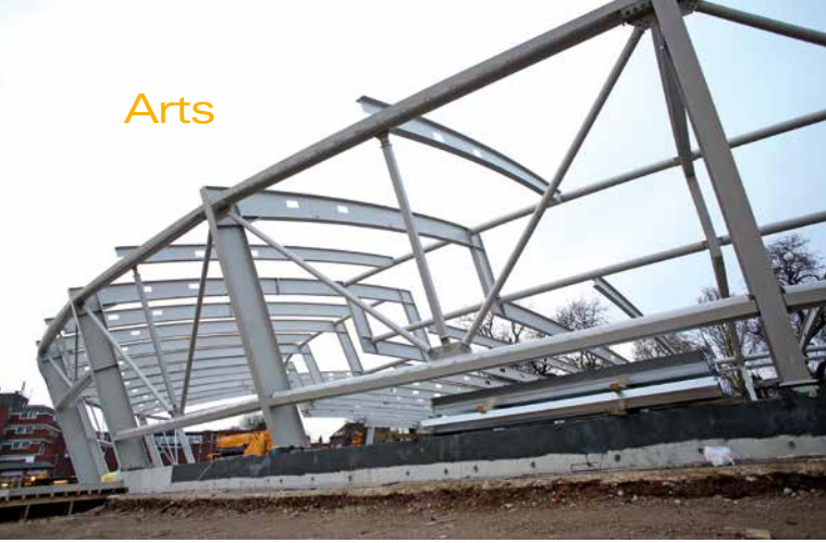
Left: The perimeter columns lean out at progressively larger degrees. Below left: The roof rafters all incorporate a step.
