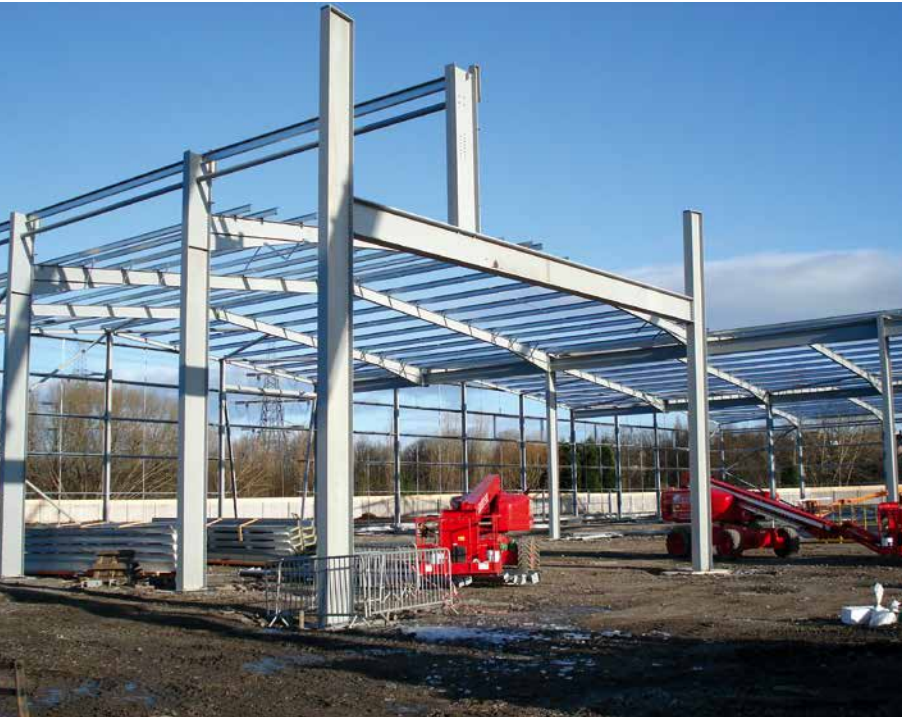
Above: The warehouse area consists of 8m wide bays.
