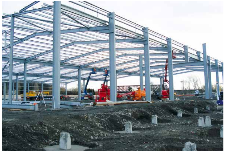
Below: The main structure sits on new 12m deep foundations.
