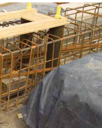
Right: The ADC will ensure all stock is stored under cover. Below: Each pile has a steel plate and a concrete pile cap with bolts to accept a column.
