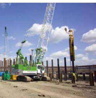
Above: Two rigs installed 316 piles for the ADC's foundations. Left: Billington Structures supplied and erected all of the steelwork for the ADC.
