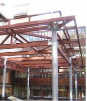
The open plan Pavilion makes use of vierendeel trusses and exposed circular columns
