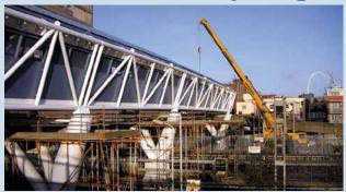
Rowecord Engineering has installed a 200t covered footbridge to serve the new Wembley Stadium. The structure forms part of a project for the London Development Agency to improve Wembley's railway station and its facilities.
