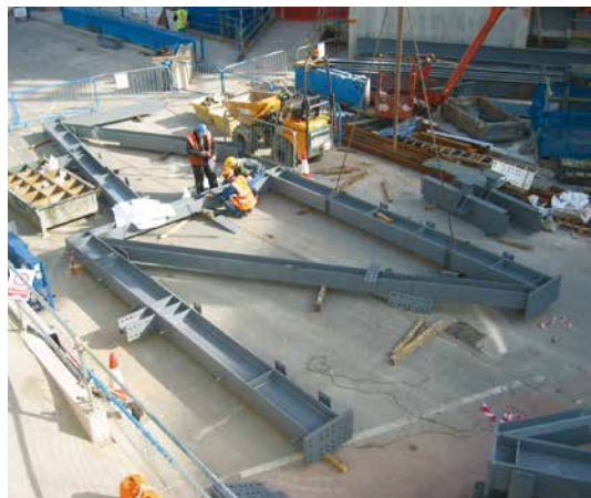
The cantilevers were assembled at the works, cut into sections for delivery to site and bolted together (above) before lifting into place (left)
