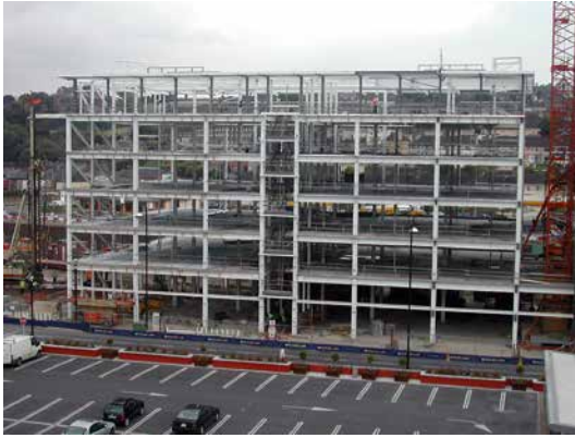
Block E is a six storey office building with retail space on the ground floor. Steel stairs were used for speed. The development is on the main Cork-Limerick road adjacent to the Blackpool Shopping Centre
