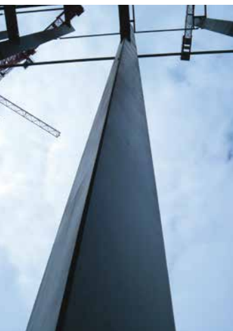
Triangular hollow section columns in the atrium rise 60m
