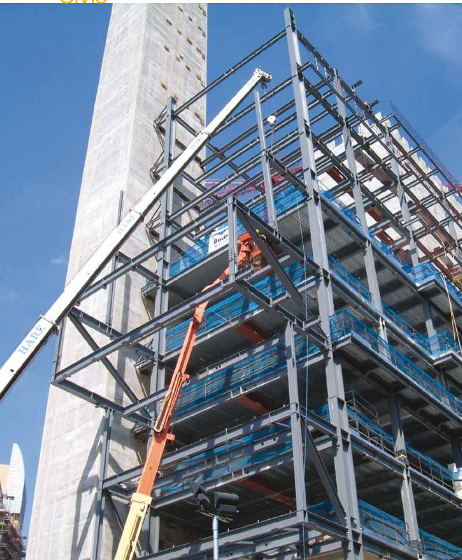
The cantilevers were assembled at the works, cut into sections for delivery to site and bolted together (above) before lifting into place (left)
