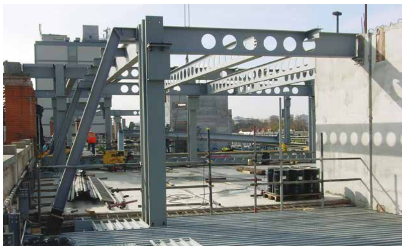
Above: most of the cladding to the rear elevation will be lifted in when the steel frame is complete. Below: a late design change to the roof was fitted into the programme.
