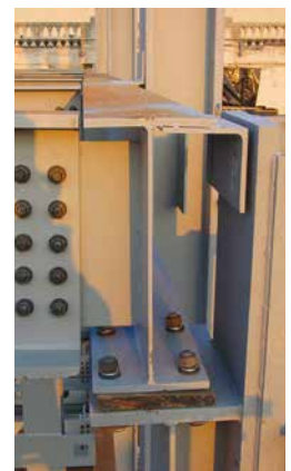
Heavy acoustic damping pads were used in the steelwork connections
