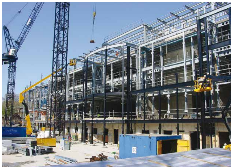
Above: most of the cladding to the rear elevation will be lifted in when the steel frame is complete. Below: a late design change to the roof was fitted into the programme.
