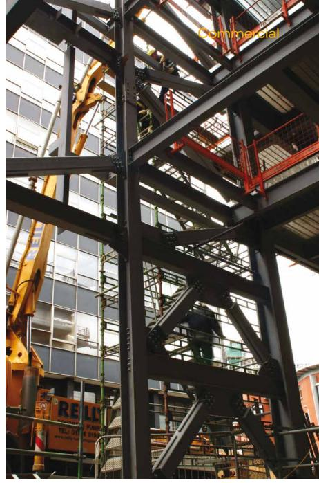
Above: Different floor levels complicated the design of columns and bracing
