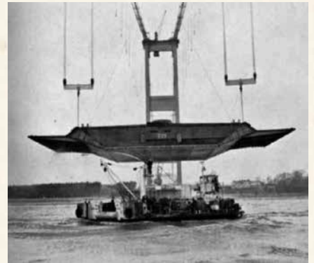
6. Washing down a deck section with fresh water.
