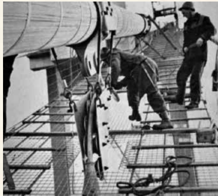
3. Feeding a suspender into position.
