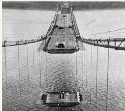
7. Deck section being lifted with bandrails and ballast tank in position.
