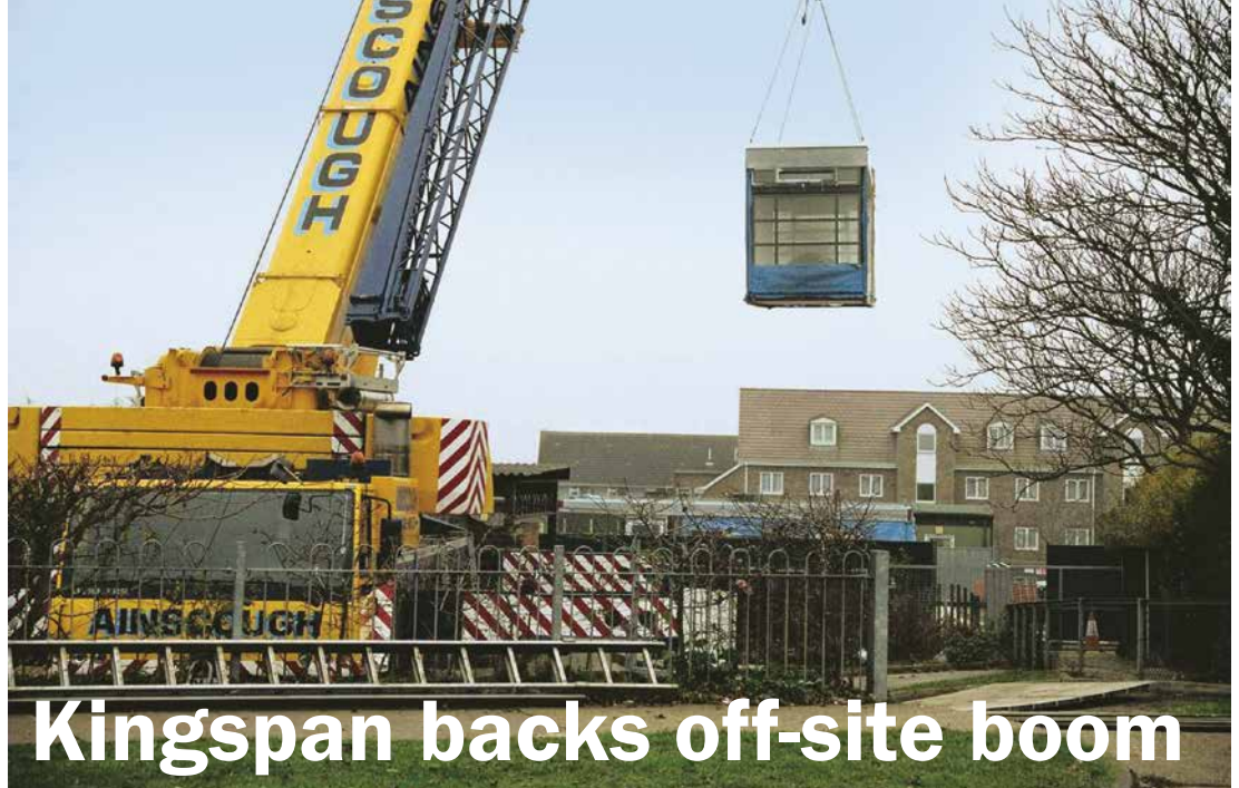
A classroom module being lifted into place at a school in Essex
