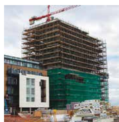
Above: Design changed from reinforced concrete to steel for speed, cost and because of more competitive market in steel.
