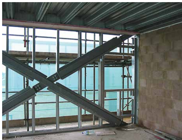
Left: Hollow section bracing members as seen from inside before wall construction
