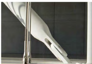
CAST CONNEX® Universal Pin Connector™ at a CHS brace member and with cast stainless steel cable fork ends in the foreground in the Whitney Museum in New York, NY
