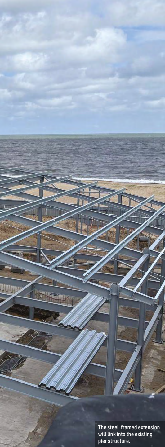
Curved cellular beams form the roof and provide the extension with its column-free space.
