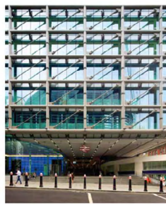
Tension system at Cannon Place, London
