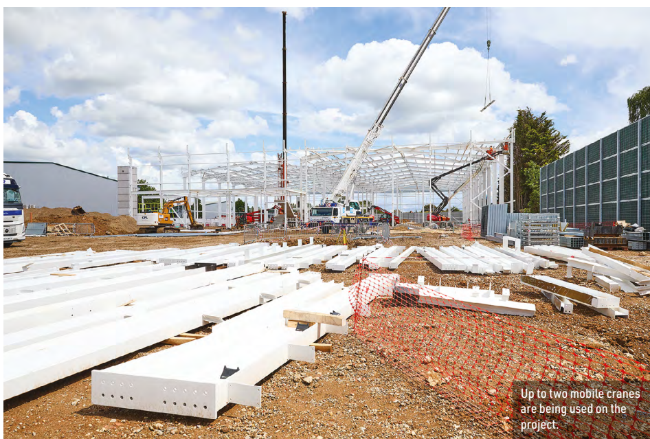
Steel was chosen as clear column-free spaces are required.
