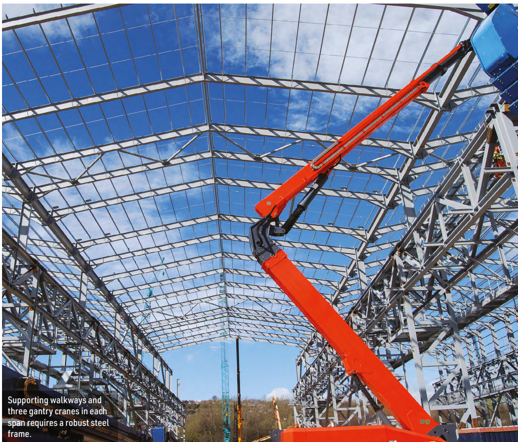
Overall, the NMS building has three internal spans, providing the necessary column-free space.
