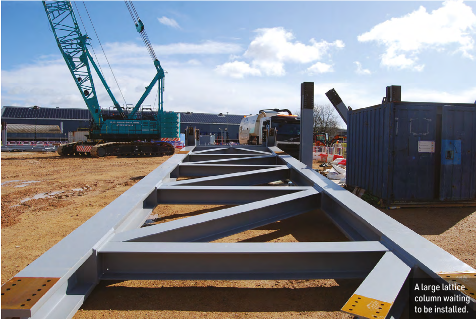
The lattice columns are connected to high-level crane supporting trusses.
