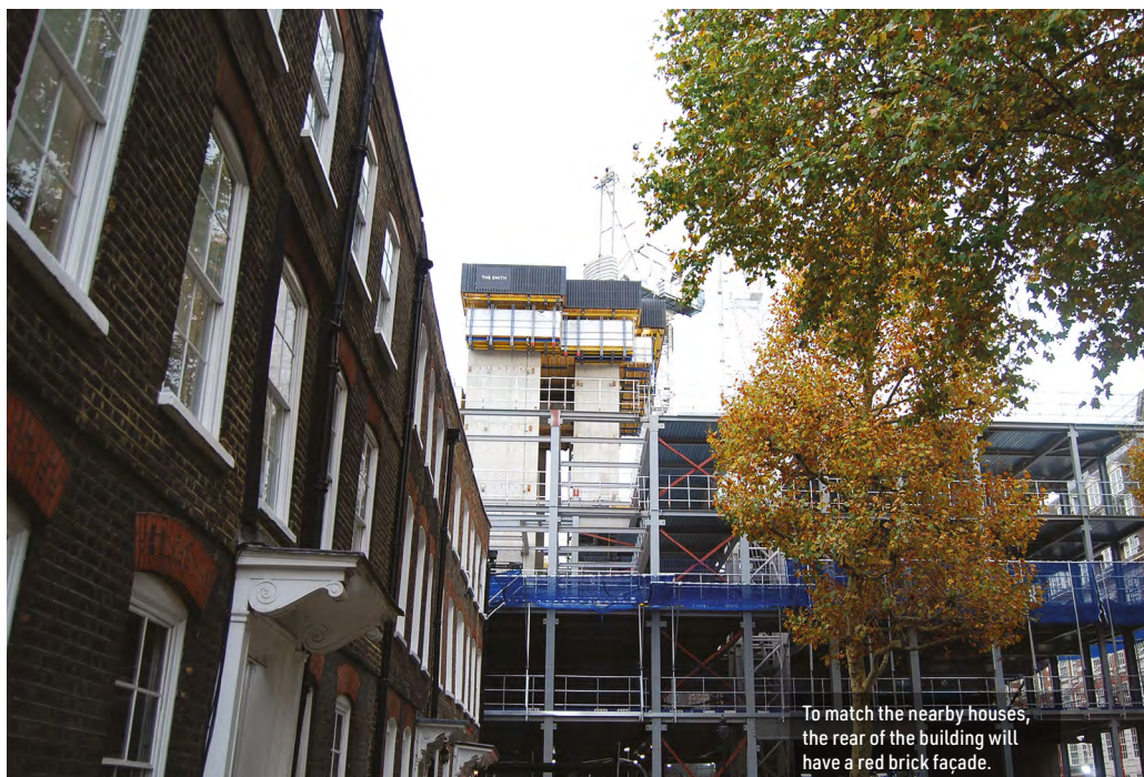
A specially designed rig, allowed the steelwork to be erected beneath the ongoing concrete works for the core.
