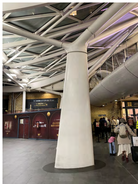
Figure 5: Cast nodes connect the 'branches' to the 'trunk' columns © John McAslan + Partners
