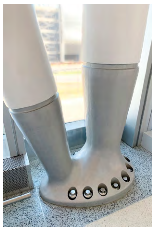
Figure 1: Example of cast steel base connection at Charlotte Douglas International Airport © CAST CONNEX
