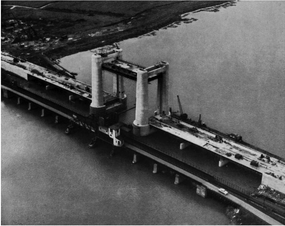
The new Kingsferry lifting bridge which provides for a vertical opening 95 ft. clear above high water. The existing river and road bridge is seen beside the new bridge.
