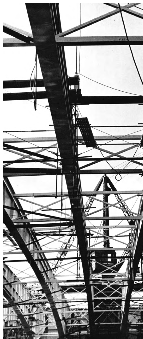
Looking up at the 270-ft. central span of Maidenhead Bridge during construction.
