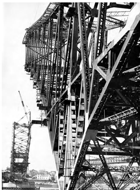
The Runcorn-Widnes Bridge under construction.
