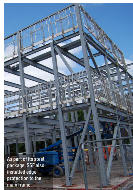
The majority of the steel frame is arranged around two rows of classrooms, divided by a centrally-positioned corridor.
