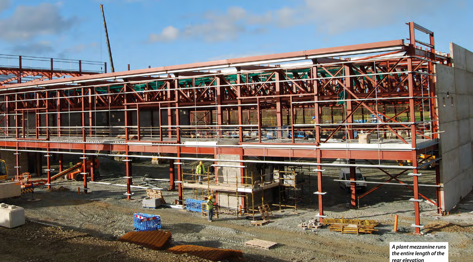
Two portal frames sit either end of the building
