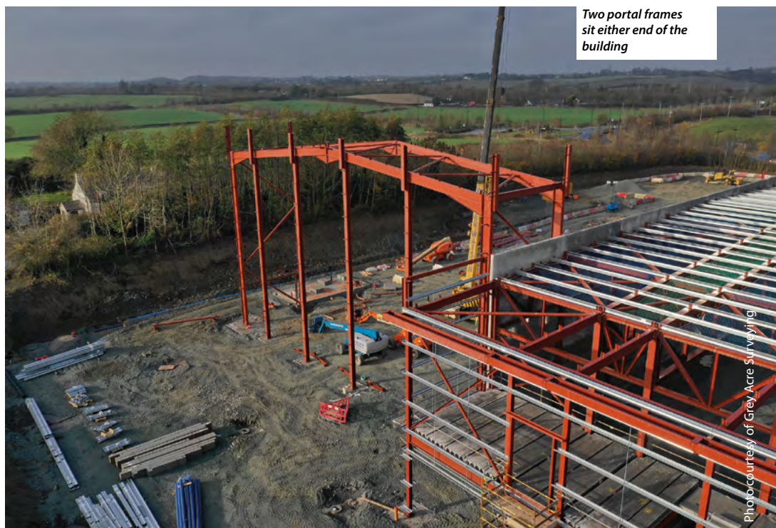
48m-long trusses form the production area
