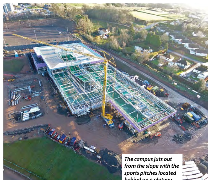
Steel erection was completed in 12 weeks
