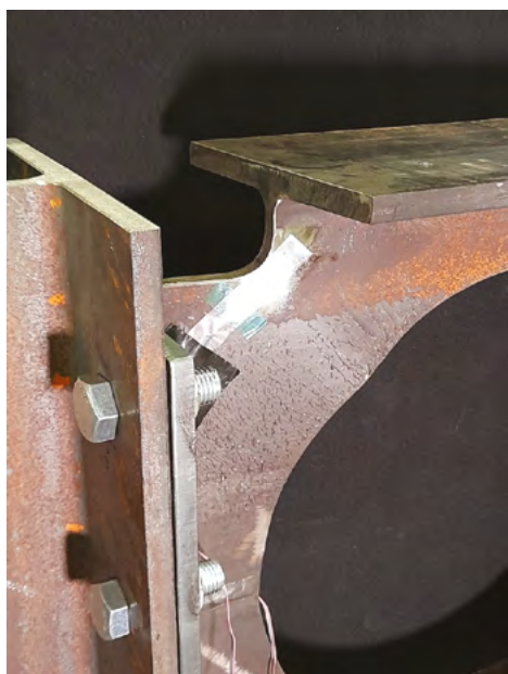
Figure 3 - Buckling at narrow end post for the notched cellular beam
