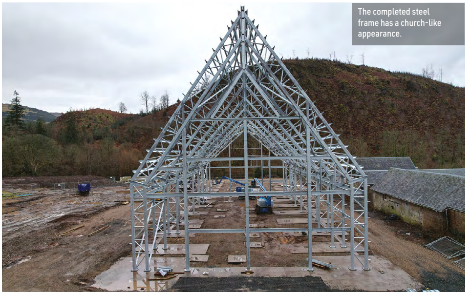
All of the steel trusses were delivered to site as fully-welded sections.
