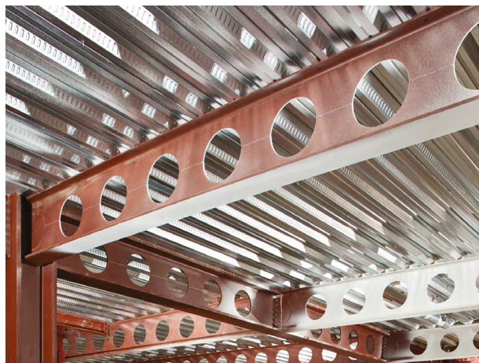
Figure 2 - Typical slender beam with infills (courtesy of Kloeckner UK Metals Westok)
