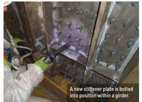
One of the original welded connections is repaired by the Taziker team.
