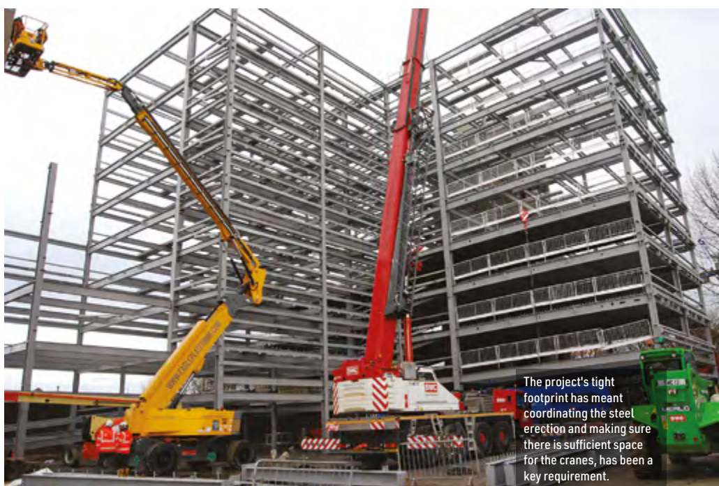
The steel frame wraps around two precast cores.
