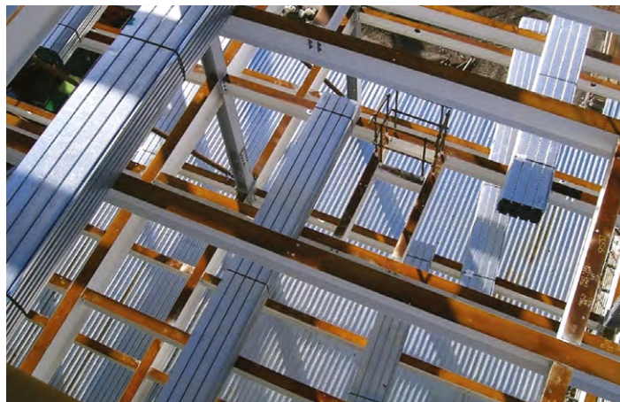
Figure 1: Decking continuous over several bays (courtesy SMD)
