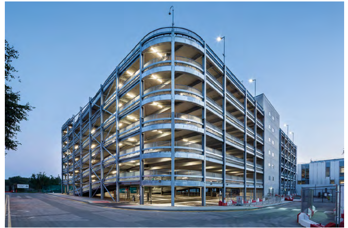
Galvanized steel carpark at Sky Headquarters (London). Photo: Philip Durrant
