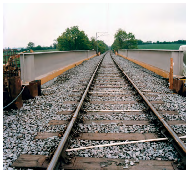
Figure 3: “Half-through” bridge
