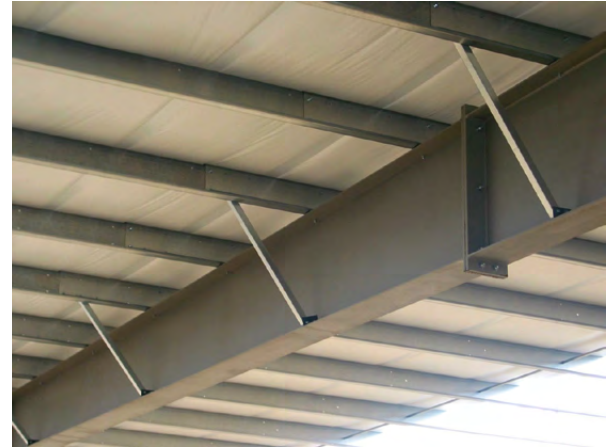
Figure 6: typical bracing to rafter
