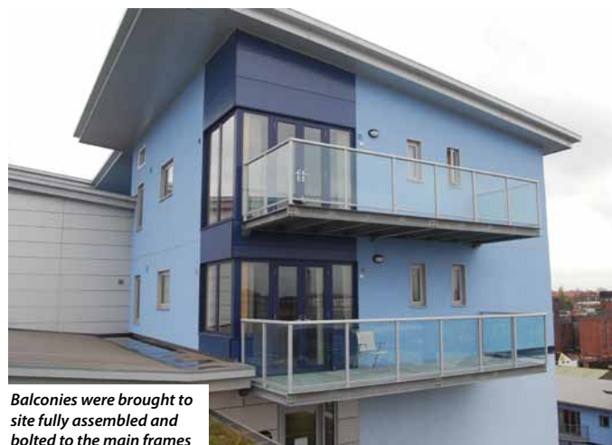
Steel frames helped the contractor with a speedy erection
