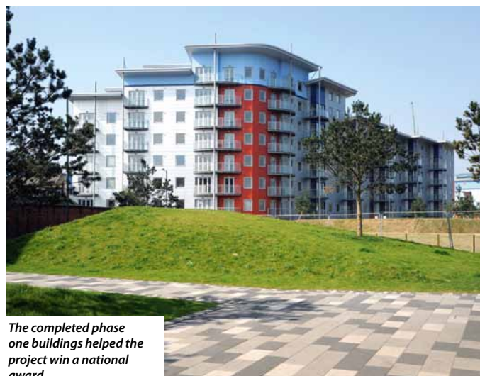
Balconies were brought to site fully assembled and bolted to the main frames
