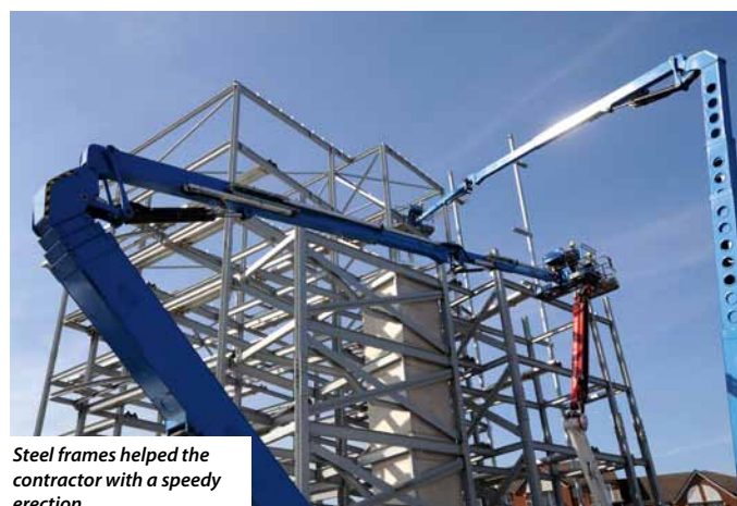
Phase two’s eight storey blocks under construction
